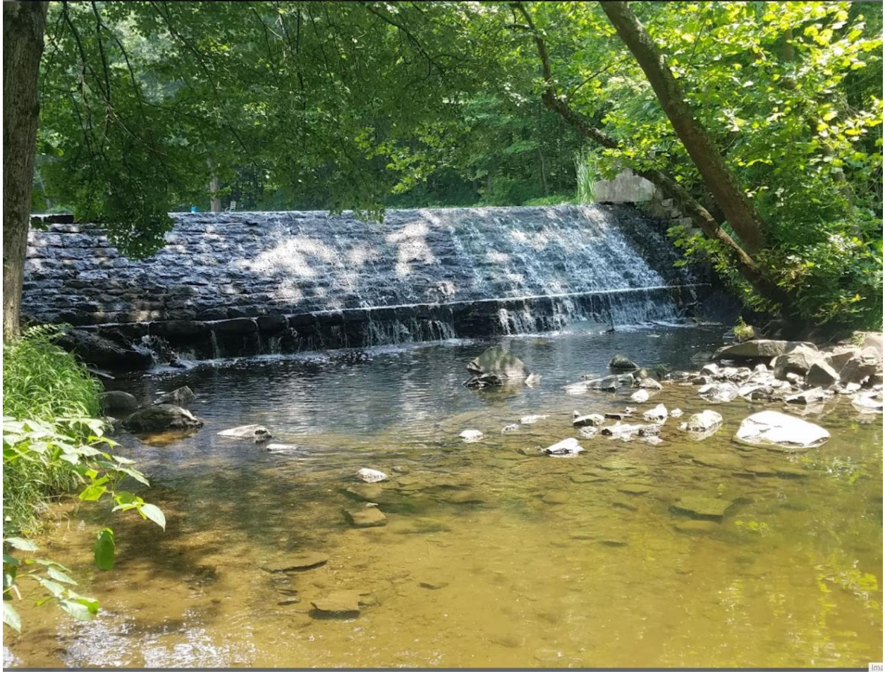
Middletown Reservoir Google Earth
